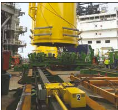
▼ The trolley system speeds up offshore wind transition piece load out: the transition pieces are positioned in the clamping frames and moved along the track.
